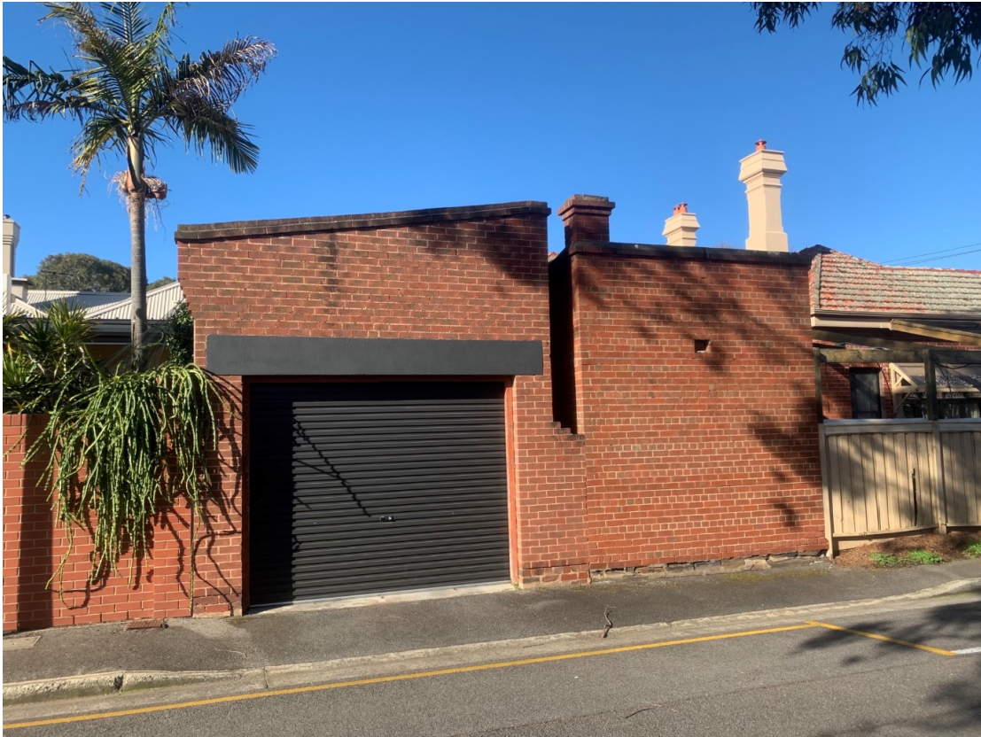
Photo 4 – Adjacent built form at rear of 84 Lefevre Terrace looking east
