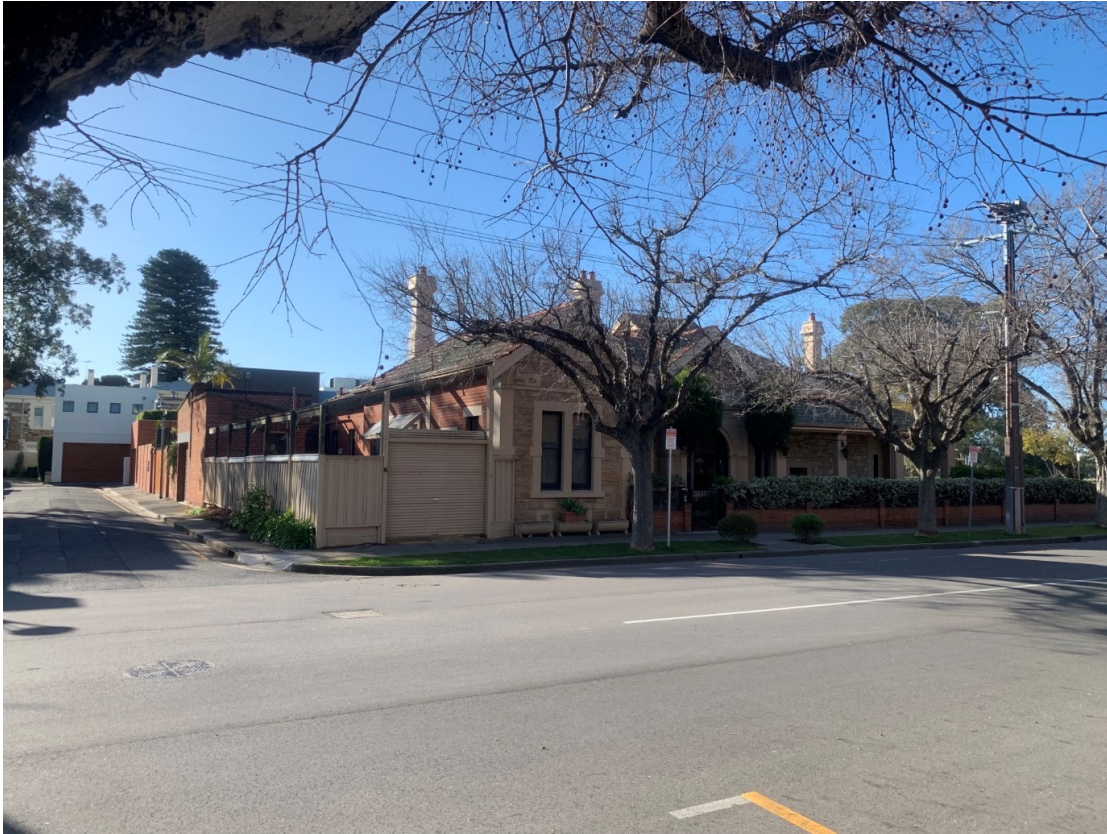
Photo 1 – Subject site looking north, viewed from Gover Street
