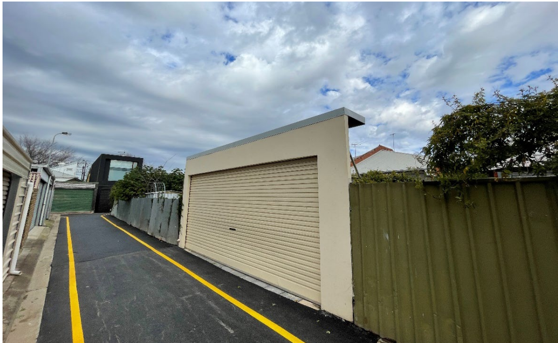
Photo 3.2 – Subject site, viewed from Dukes Lane looking west
